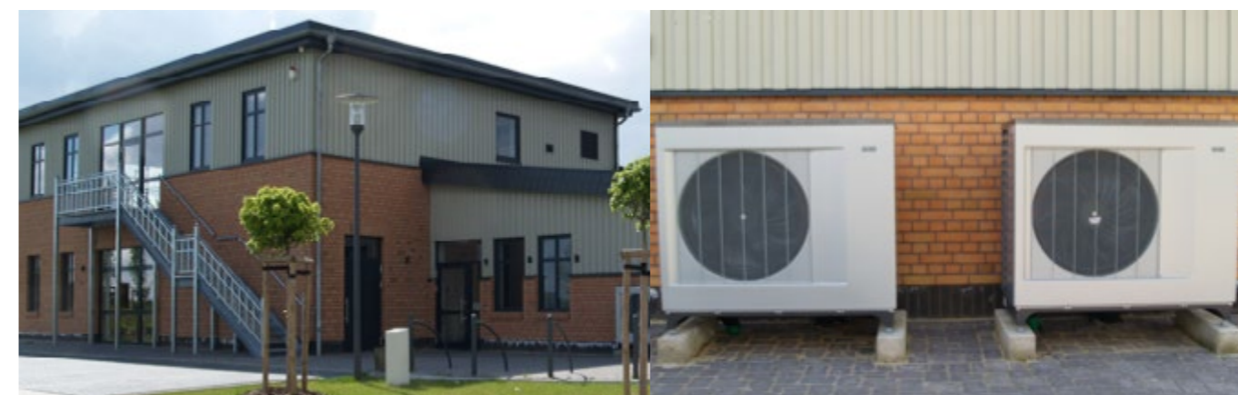
Figure 13: Volunteer fire station in Lachendorf
